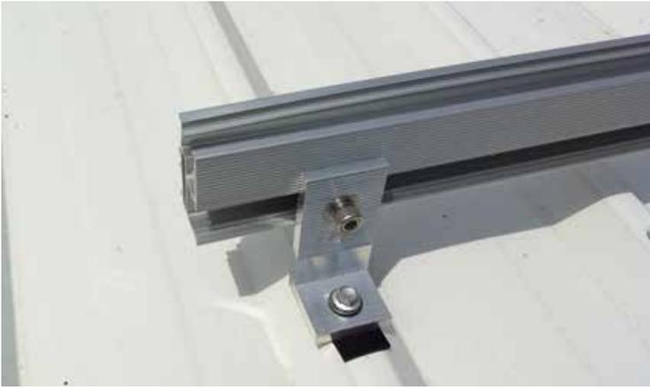
All fixings securely tightened (note black strip to separate different metals)
